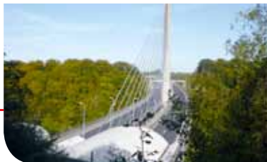
Pont Victor Bodson, Hesperange, env. 6 km Brücke Victor Bodson Hesperingen, ca. 6 km
